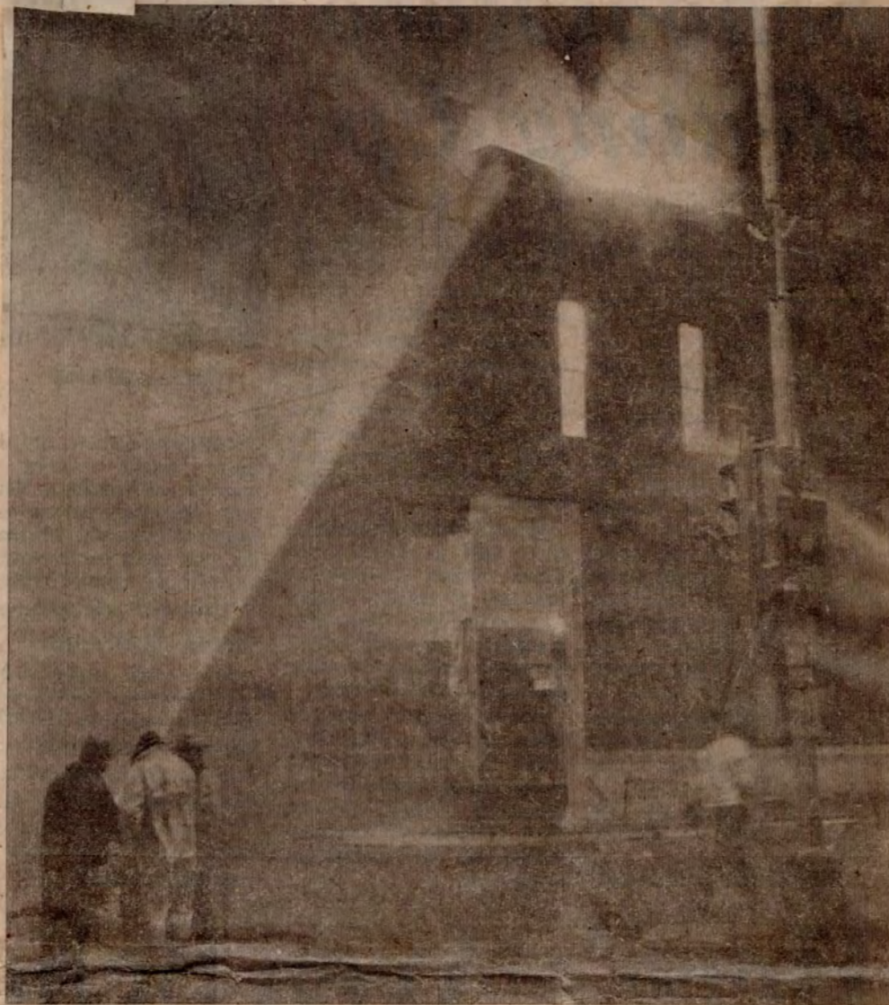
Fire Guts Businesses
