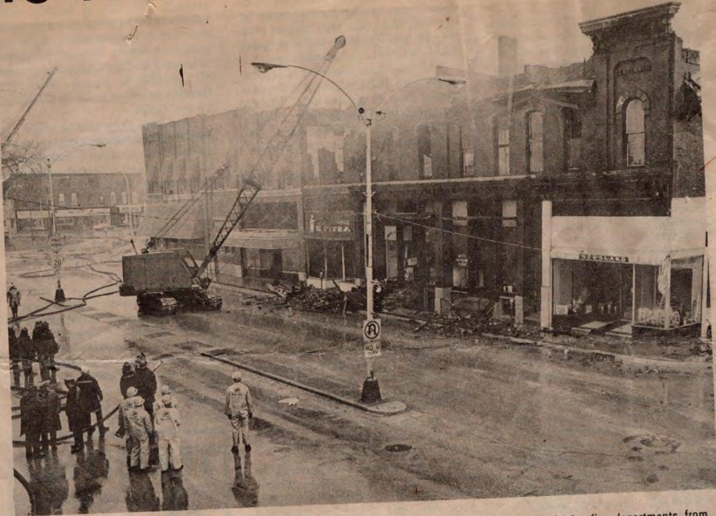
DAMAGE HAS BEEN estimated at more than $1 million as a result of an early Thursday fire which gutted almost a block of Main street business houses in downtown Monmouth, Ill. The blaze was fought by fire departments from Galesburg, Alexis, Roseville and Monmouth. (Hawk Eye photo by John Gram)
